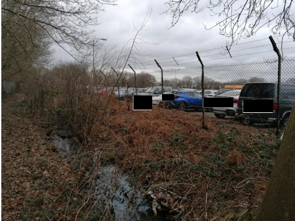
Above (February 2024) and Below (September 2021):Section of Footpath 360Sy (between the footbridge looking north west). Note poor condition of drainage ditch and limited path width due to car park fences running parallel to path and ditch. Ditch not readily visible in summer autumn.
